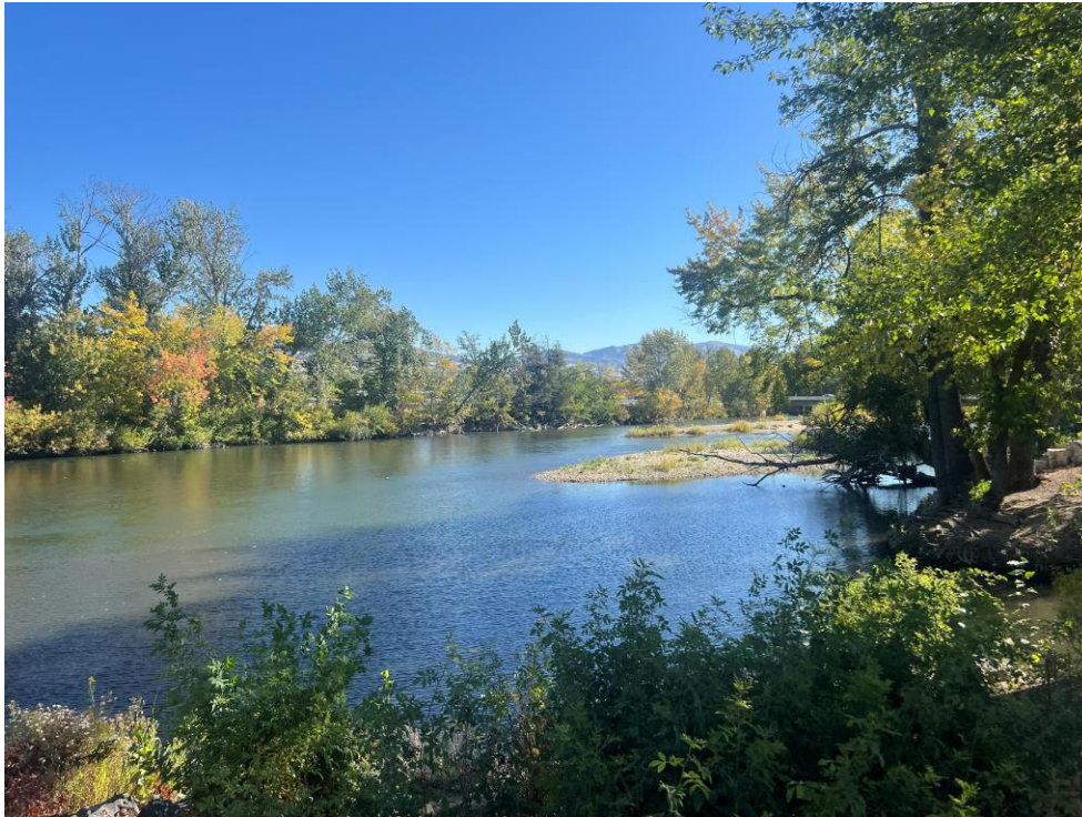
Looking northwest from W Main St Bridge at approximate area where bridge will span.
